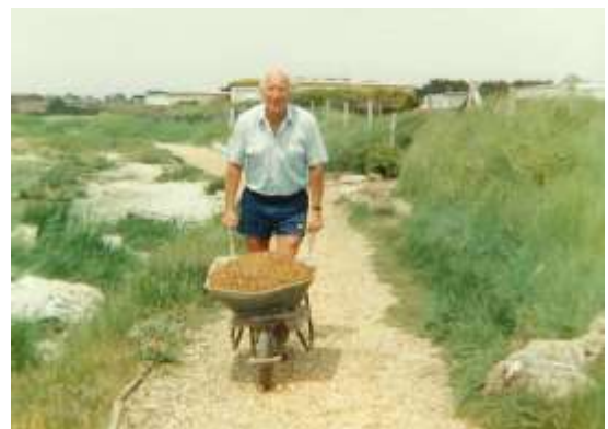
The late Bill Smith laying gravel
