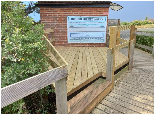
The new raised decking.
